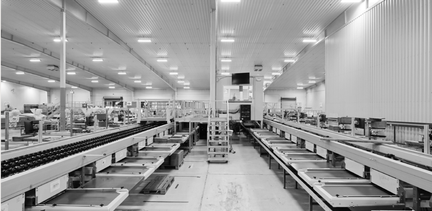
Interior of the Turners and Growers facility, Nelson
