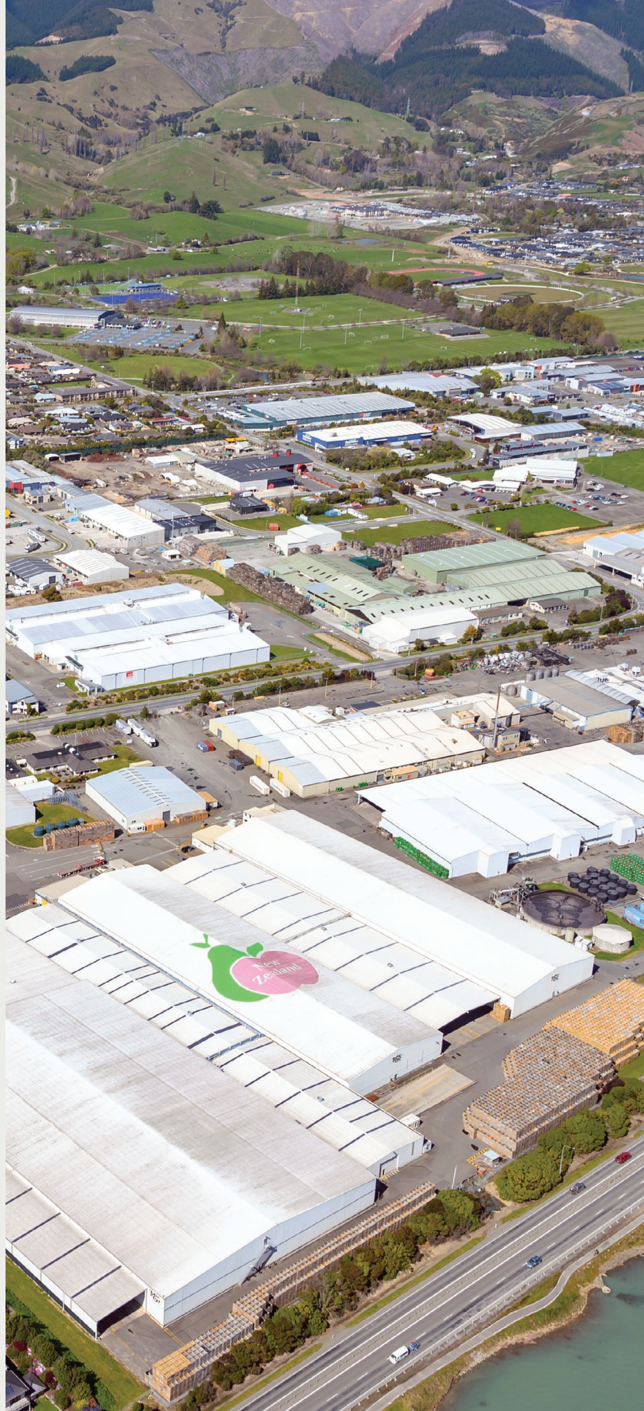
Aerial view 484 Nayland Road, Nelson
