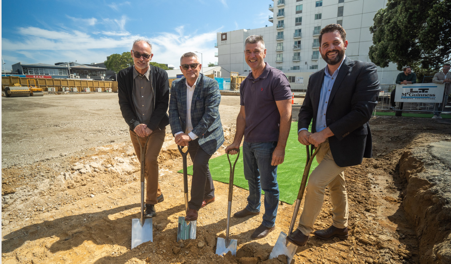
Left to right: Willis Bond Managing Director (Funds & Finance) Wayne Silver, Tauranga City Council Commissioner Bill Wasley, Tauranga City Council CE Marty Grenfell, and LT McGuinness Director Matt McGuinness breaking ground at 90 Devonport Road
